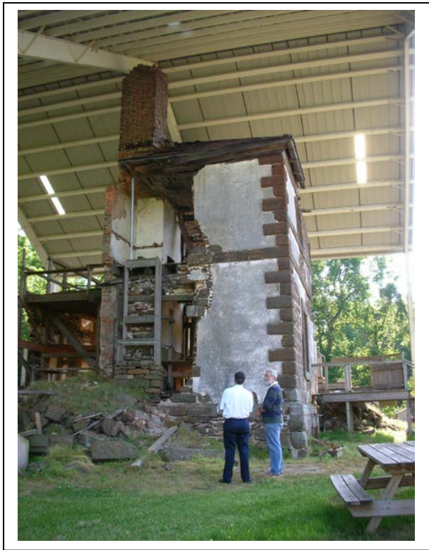
Fig. 28, 29: Macfarlane and Phillips conferring about details for the East wall enclosure. As with most projects that involve unique detailing, it is best to do much of it on site. The right view shows the Plexiglas enclosure in place before the shading film detailing was applied. Although the glare provides a presence for the glass skin it does not visually overpower the original structure. It does temporarily mask the interior which aids in understanding the form of the building.
