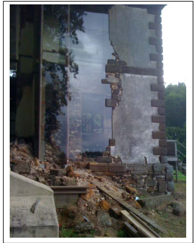
Fig. 28, 29: Macfarlane and Phillips conferring about details for the East wall enclosure. As with most projects that involve unique detailing, it is best to do much of it on site. The right view shows the Plexiglas enclosure in place before the shading film detailing was applied. Although the glare provides a presence for the glass skin it does not visually overpower the original structure. It does temporarily mask the interior which aids in understanding the form of the building.
