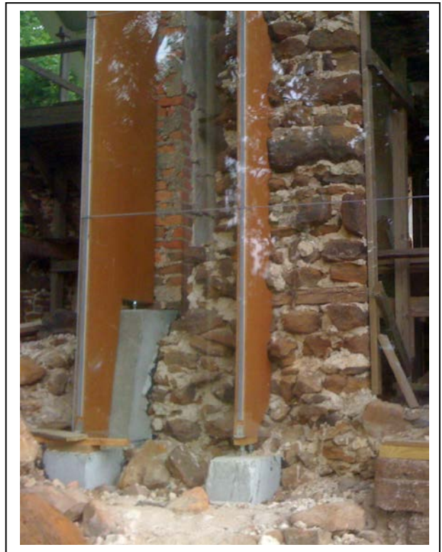
Fig. 30, 31: When not standing where the glare is brightest, one can see the plywood fins. At the right the cast concrete bases for the fins are easily visible – a more elegant solution can be found. There is a sheet of plastic between the concrete and the historic masonry as a bond breaker. Interpretively this relationship with the glare also allows one to see the interior makeup of the building and how it goes together (form/detail).
