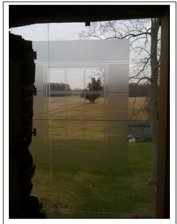
Fig. 32, 33: These views show the appearance of the shading film detail from the exterior and the interior.
