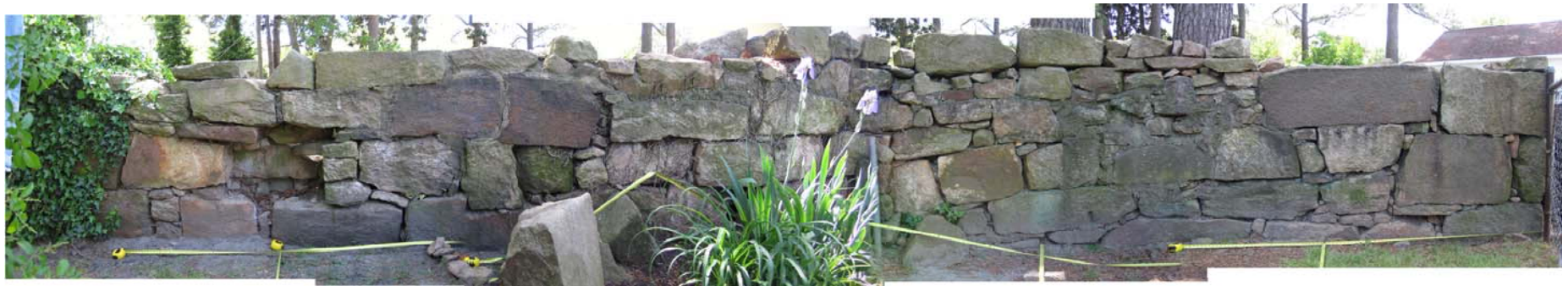
WALL VIEWED FROM OUTSIDE CEMETERY
